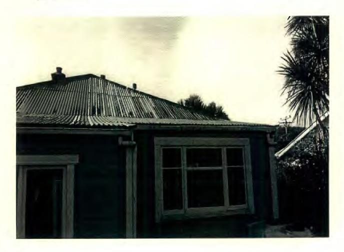
This photo shows the roof that is supported by the new beam. The beam is on the line of the change in the roof angle. The main window shown is the kitchen window.
